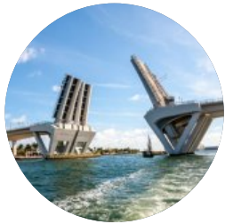
BRIDGES & MOVABLE STRUCTURES
